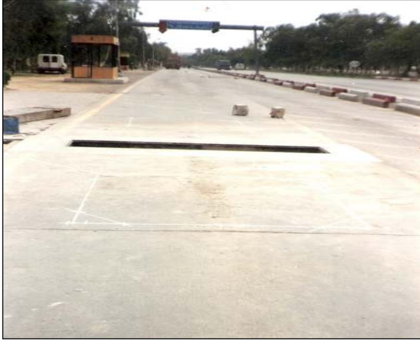
Slow Speed Weigh In Motion Scale (SSWIM) at Sangjani National Highway N-5
